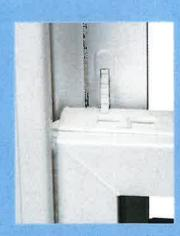
Easy-to-use, low-profile vent latches limit how far the sashes can open. Windows can still be vented but limited to help deter entry.
