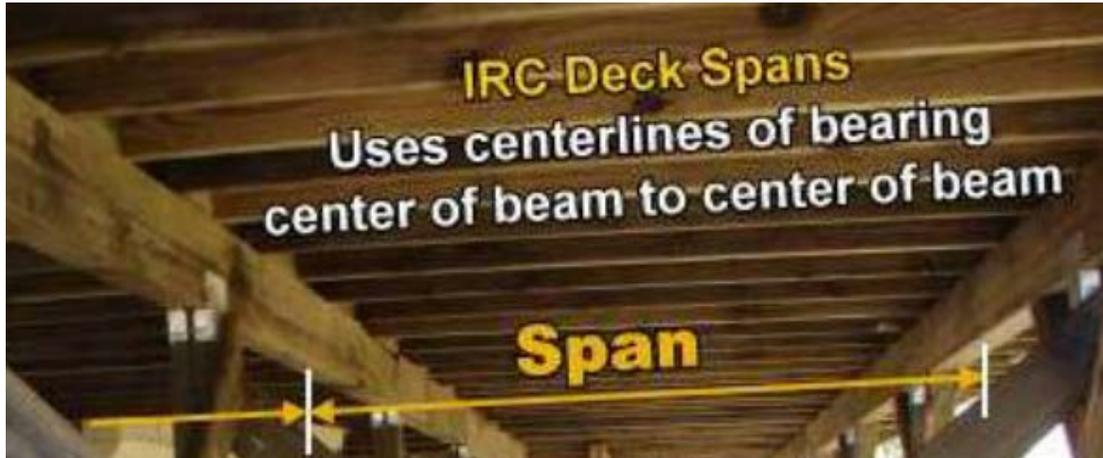
DECK BEAM SPAN LENGTHS<sup>a, b</sup> (ft. - in.)
