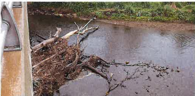
Removing debris from streams.
