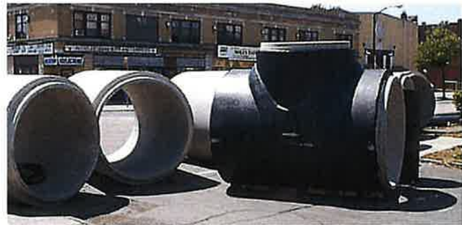
Installing storm sewers. Source: http://www.erdmananthony.com/ProjectPortfolio/Detail.aspx?id=41
