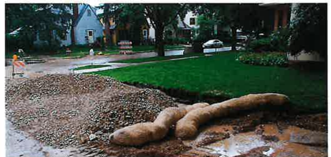
Upgrading local drainage. Source: http://saveourstream.blogspot.com/p/green-infrastructure.html
