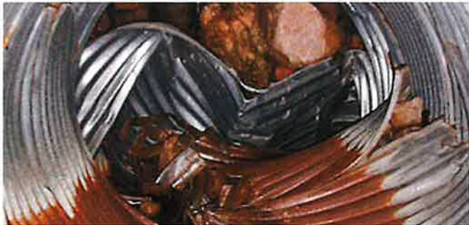
Replacing failing culverts. Source: www.newnhamfarms.com
